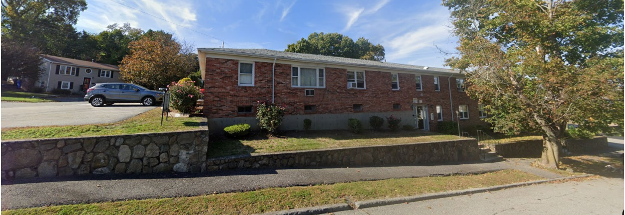
View from Dart Street, Unit 21 conversion proposed for bottom left of building (Google Street View, Oct 2022)
